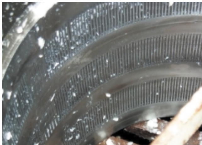
5. No evidence of PSA buildup on screen interior
