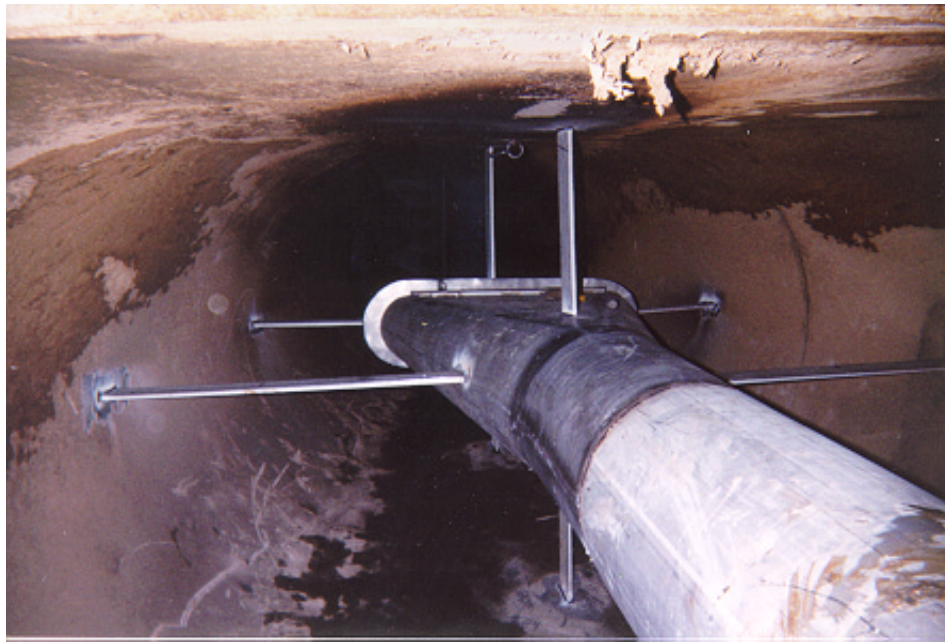
Figure 10. Mixing wedge installation photograph.
