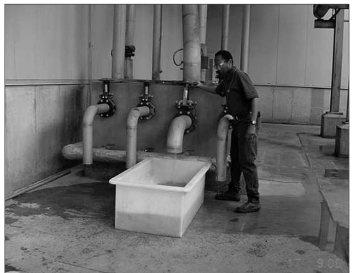
4. The author dumping flows from back of seal pit weir box.
