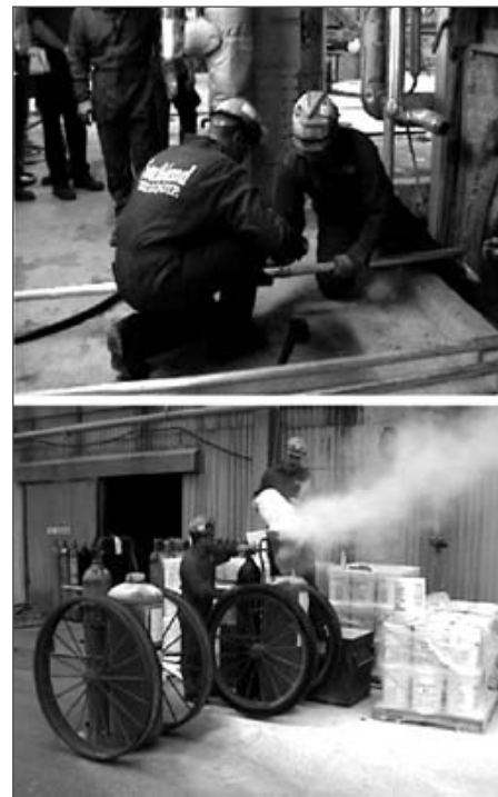
3. Workers preparing the lance and the canisters for injecting bicarbonate.
