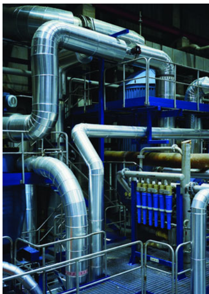
Chemithermomechanical pulp plant.
