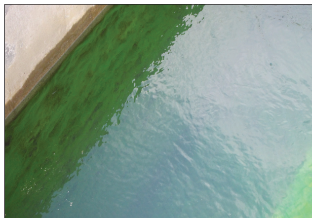
5. Growth of green algae on the wall of a channel taking recycled water from the cooling towers.
