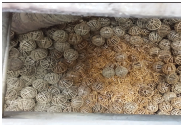
6. Broken tellerets in the TRS sump packed bed.
