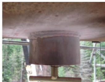
(e) Final installed socket for the gas cartridge
