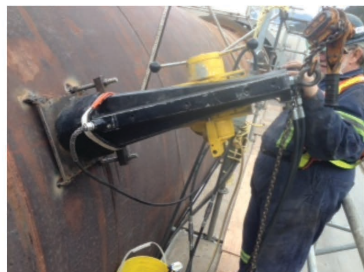
(a) Electromagnetic drill press used to machine hole in the kiln shell
