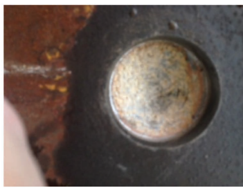
(b) Access hole used for the gas cartridge (refractory still in place)
