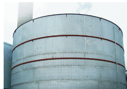
Constructed in 2004, one of the first process tanks using lean duplex 1.4162/2101. It is at Stora Enso's mill in Imatra, Finland.
