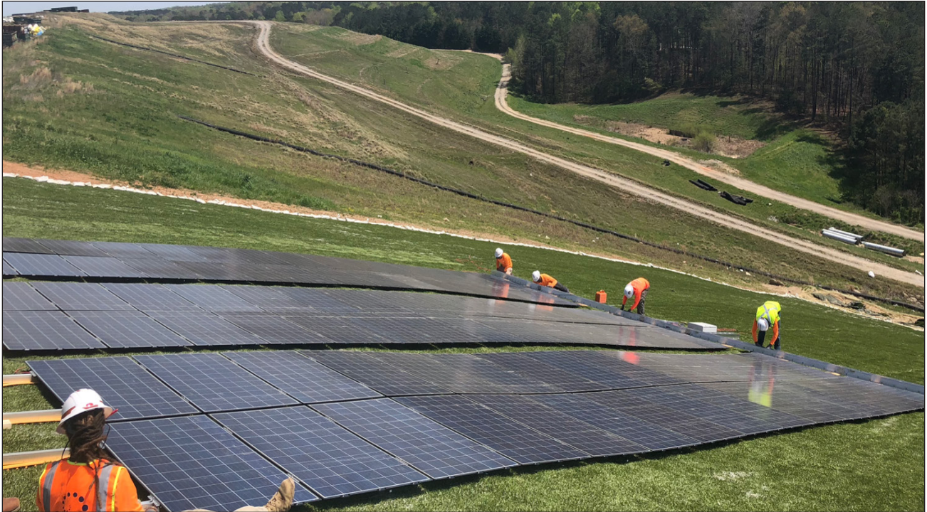
7. Installation of solar system on a landfill slope.
