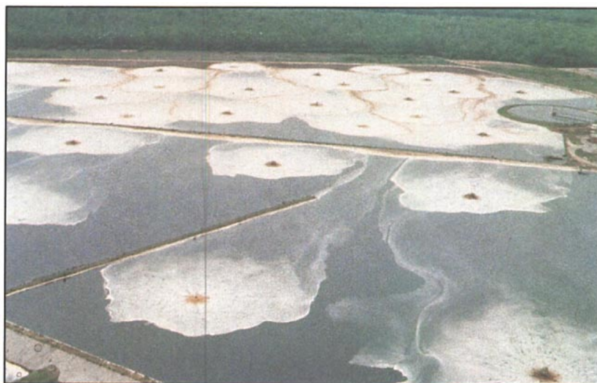
1. Pulp mill bioponds. Effluent treatment has been a stronghold of biotechnology for many years. New research may lead to improved methods for removing color and reducing AOX.
