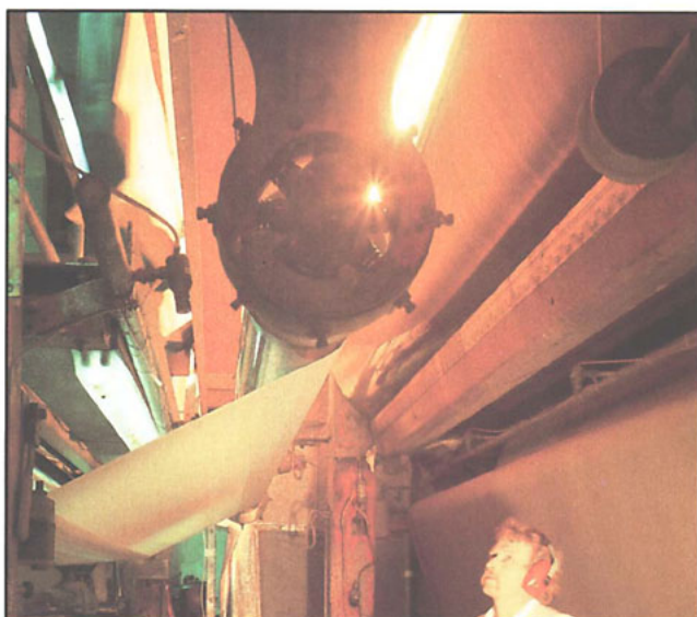
4. The infrared dried system on PM No. 5 regulates the cross profile moisture.
