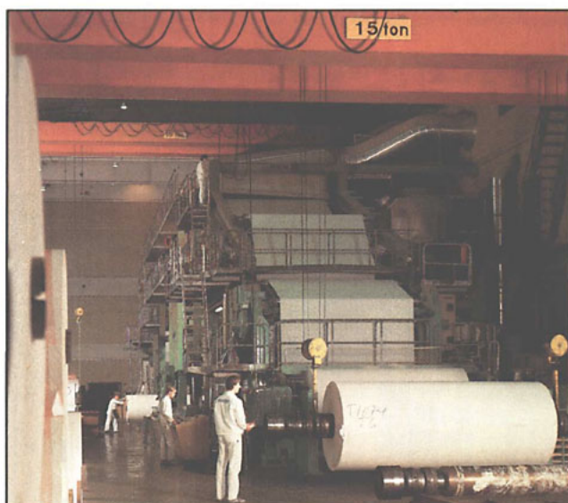
6. The existing off machine coater was made by Karlstads Mekaniska Verkstad.
