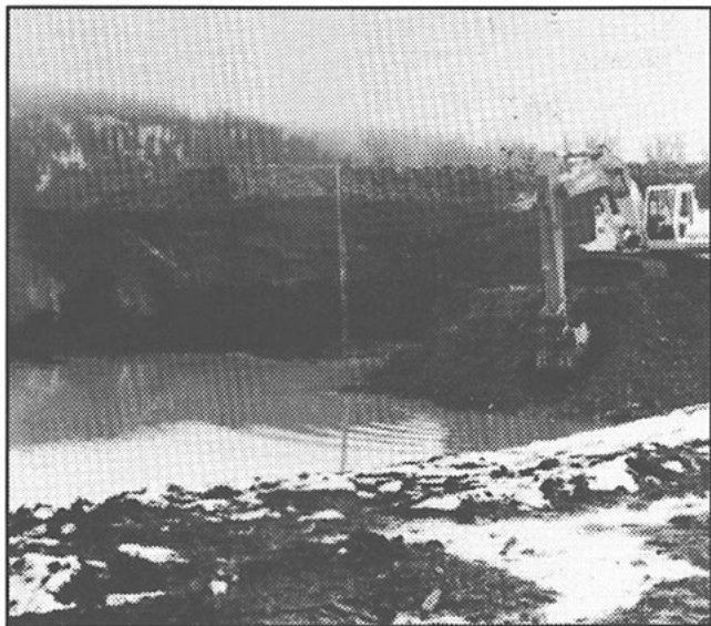
5. Rocks are placed in liner for later treatment.
