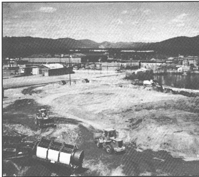
6. One-acre land treatment unit prior to placement of contaminated soil
