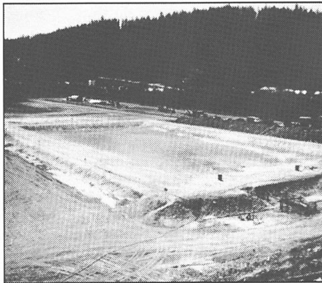
6. One-acre land treatment unit prior to placement of contaminated soil
