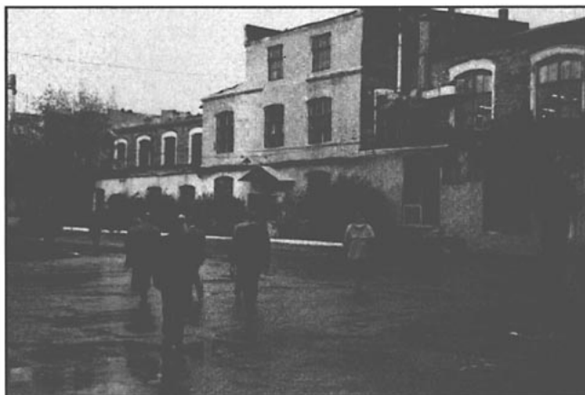
Buildings of the Krasnogorodsky mill complex
