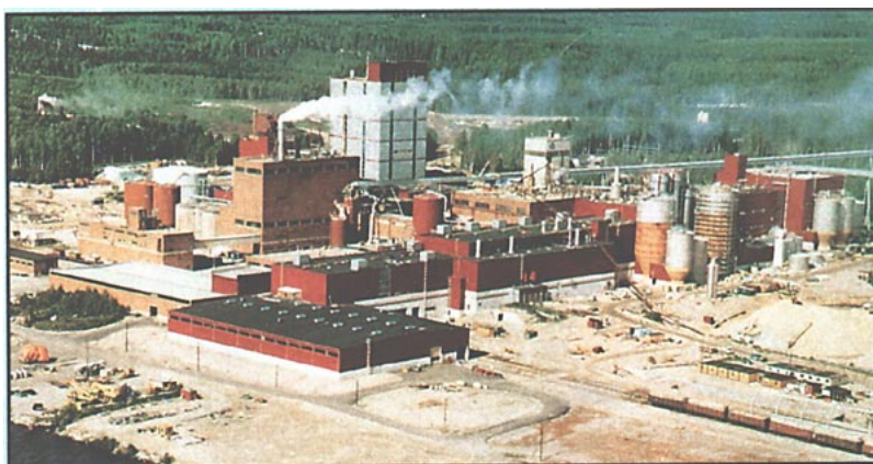
Hot liquor accumulators in front of the SuperBatch digester plant
