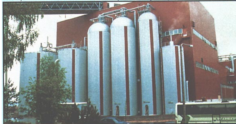
Displacement presses for post-oxygen washing
