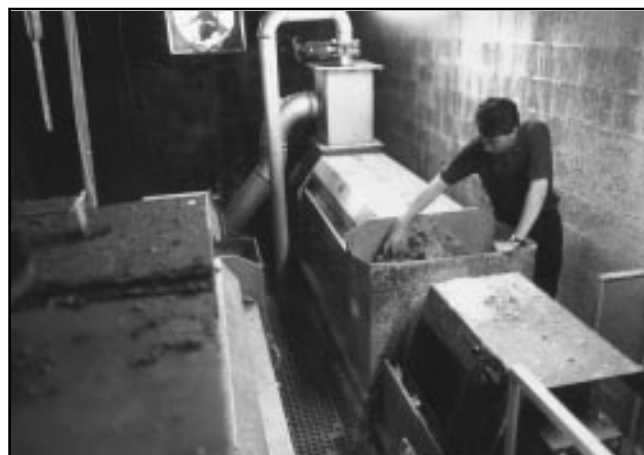
2. Screw press installation at the mill has facilitated sludge removal.
