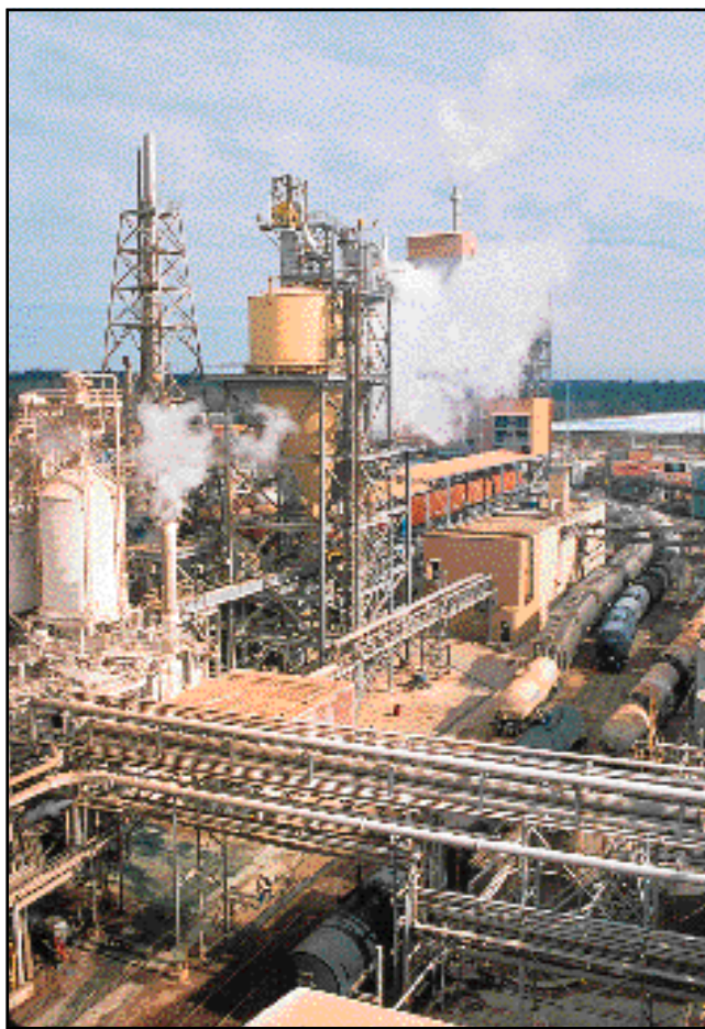
1. South view of lime kiln
