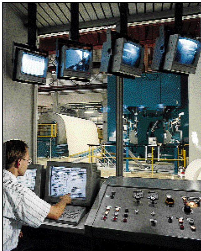
4. PLC in the mill
