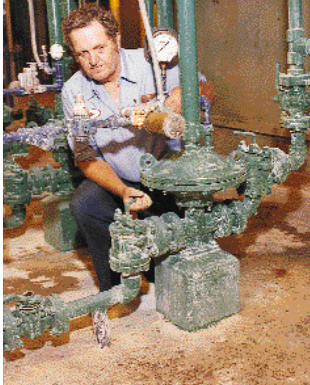
The ODS pump is a single-action reciprocating pump used in green liquor applications in the plant and also in the wastewater treatment area for sludge handling. (Photo courtesy Dorr-Oliver.)
