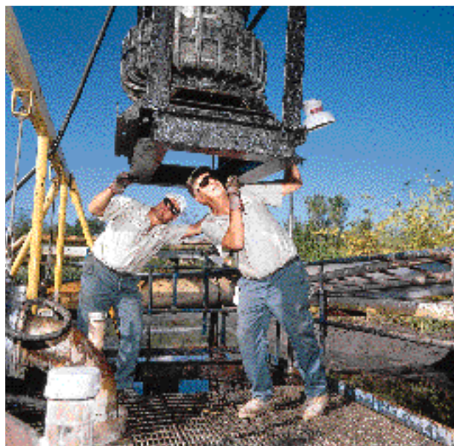
An air-actuated pinch valve. (Photo courtesy Red Valve Company.)
