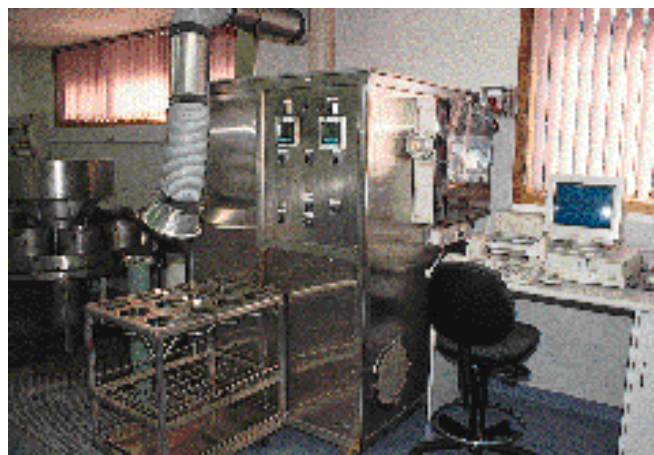
One of the laboratory work stations at Ridgley, with an "elephant trunk" exhaust tube extending from the ceiling
