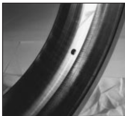
15. Corrosion from excessive wash down
