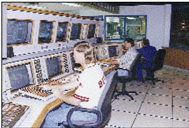
The process control room
