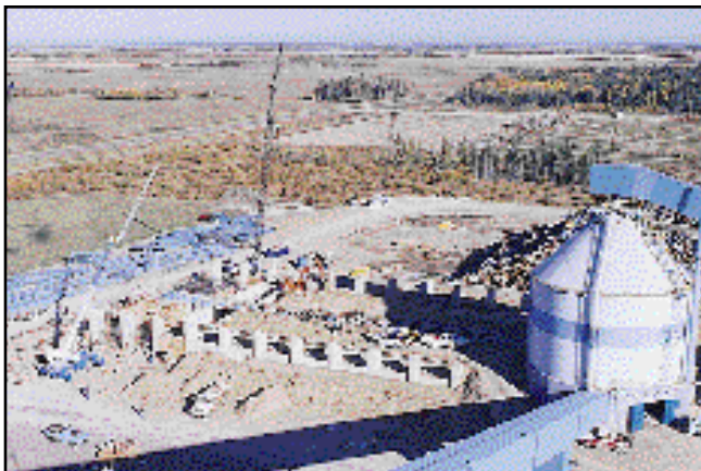
A-frame chip storage under construction
