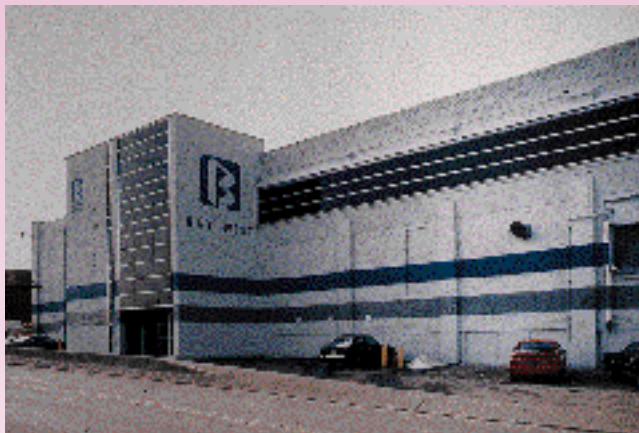
Bay West paper mill, Middletown, OH
