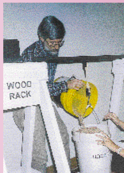
(below) The "Wood Rack." Terry Conners adds weight to the dogbone-shaped pine sample being tested. After the sample breaks, the rocks will be weighed on a small scale.
