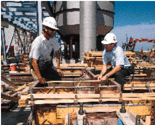
BE&K employees and subcontractors worked together to build the mill.
