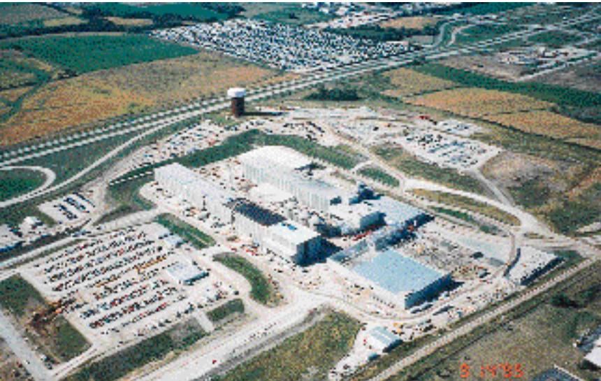
Cedar River during construction of the No. 2 linerboard machine
