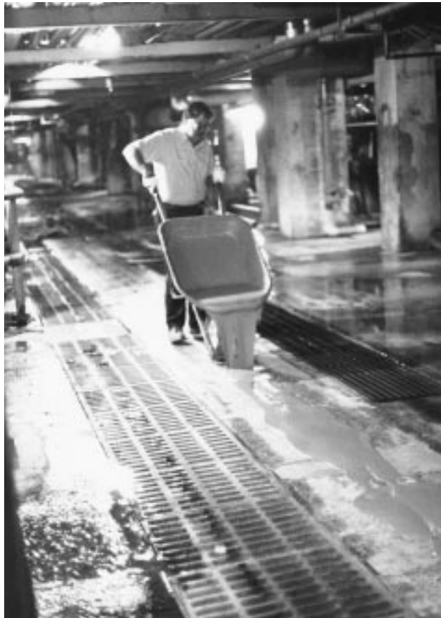
2. The floor topping is smoothed with a trowel to a depth of 250 mils (0.25 in.). With a compressive strength of about 12,000 psi when cured, this surface can withstand extremely heavy loads. It also resists wear, abrasion, and moisture.
