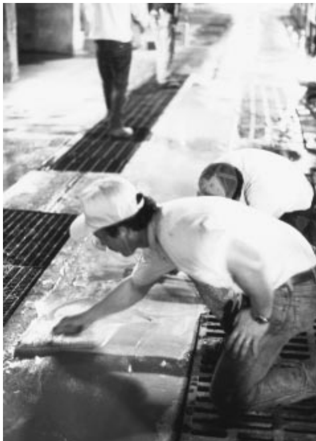
1. A resin-rich flooring is poured onto a previously prepared section of floor between two floor drains and then smoothed with trowels. This area has been cleaned to remove loose concrete and to create a surface profile for better adhesion of the flooring. Although surrounded by wet floors and high humidity, the new floor topping adheres well to this still-damp section.
