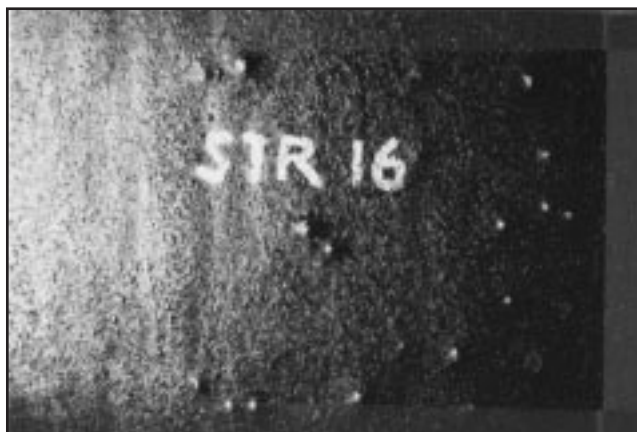
6. "Spikes" on the wall of a continuous digester, between the cooking and extraction screens
