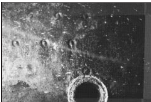
7. Erosion-corrosion behind an extraction screen
