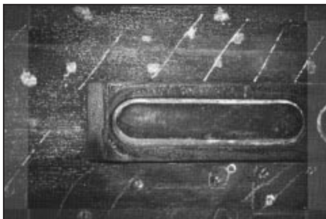
13. Anodic protection with wall-mounted cathodes
