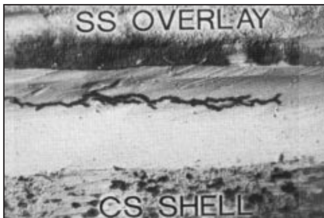
15. SCC in the carbon steel at the edge of the stainless steel weld overlay band in the impregnation zone of a continuous digester
