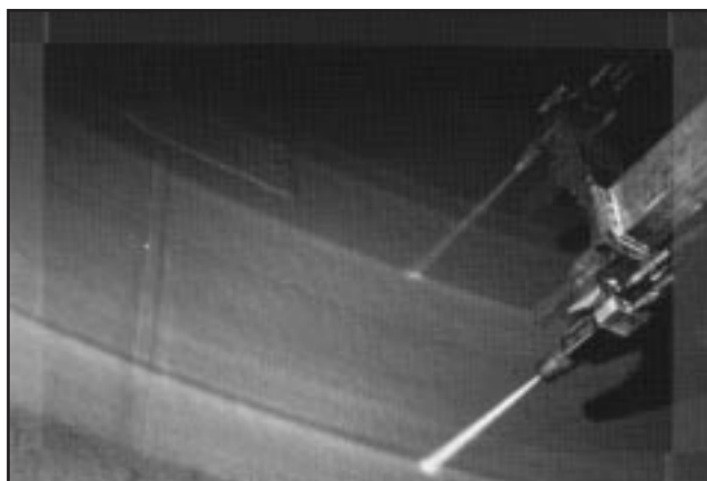
16. HVOF thermal spray being applied by a robot arm in the wash zone of a continuous digester
