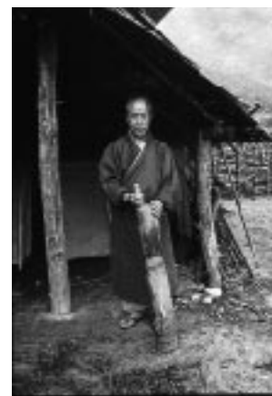
Sikkim - Churning to disperse beaten fibers in water before forming (Field)
