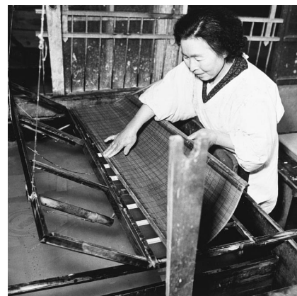
Japan - Laying a bamboo screen on the mould (RCWAMP)
