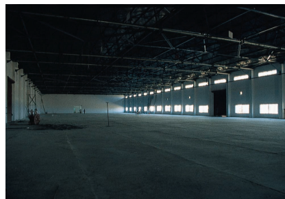
The warehouse and shipping area
