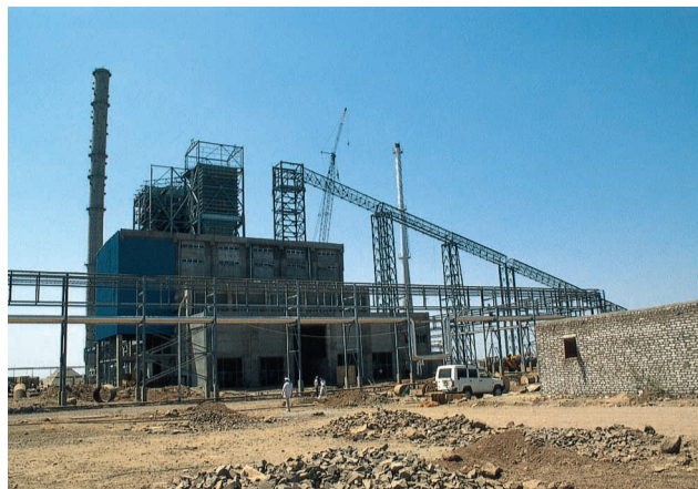
The boiler complex under construction
