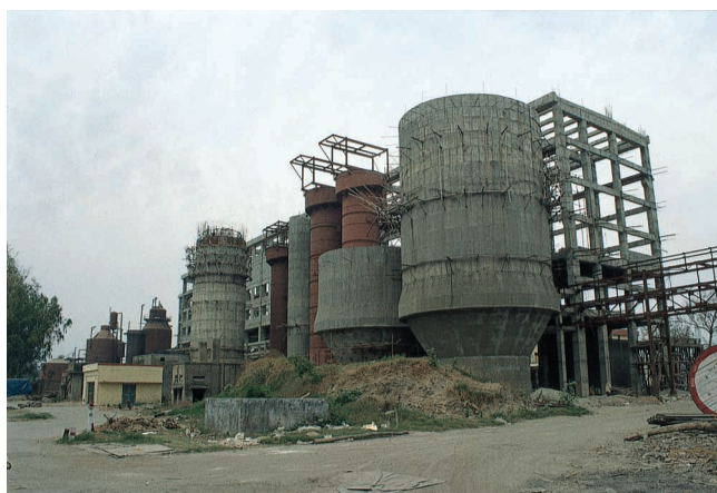
Construction of the new pulp mill at Shree Gopal
