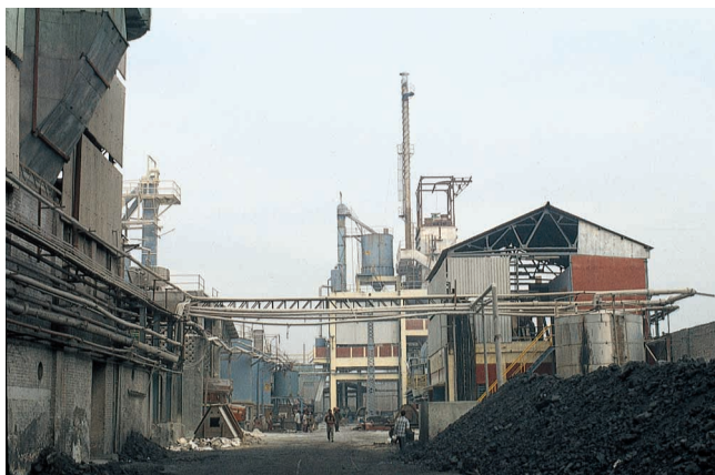
Coal storage and the recovery area at Star
