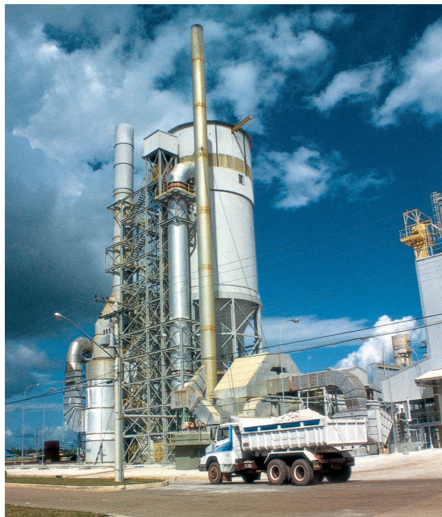
RCC's kaolin processing plant
