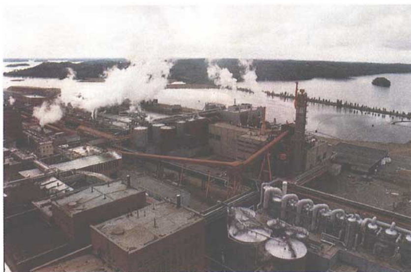
The Kaukopää mill sits between Lake Saimaa and the Russian border
