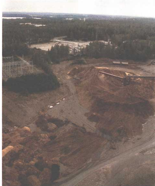
Wood yards, rejects and a power station at the Kaukopaa mill
