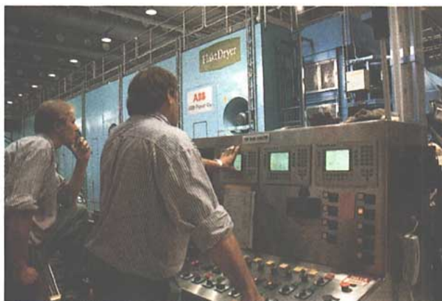
Manning the controls for the pulp dryer section at Kaukas
