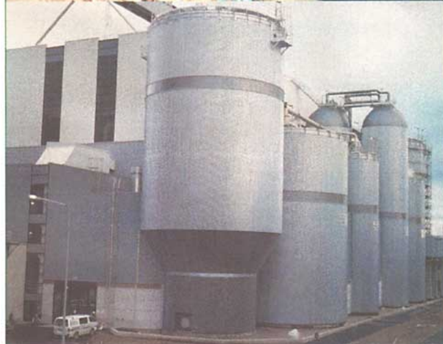
The Camura GentleSlice™ chipper (top) and SuperBatch™ cooking plant at the Kaukas mill (photos: Sunds Defibrator)
