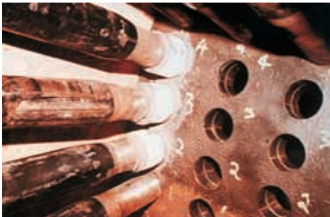
2. March 1994 installation of ceramic shields during generator tube installation
